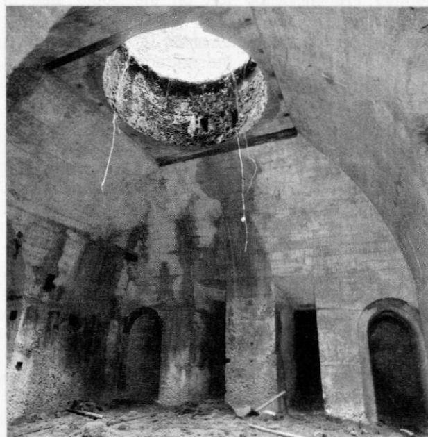
The underground chamber beneath No. 1 turret
